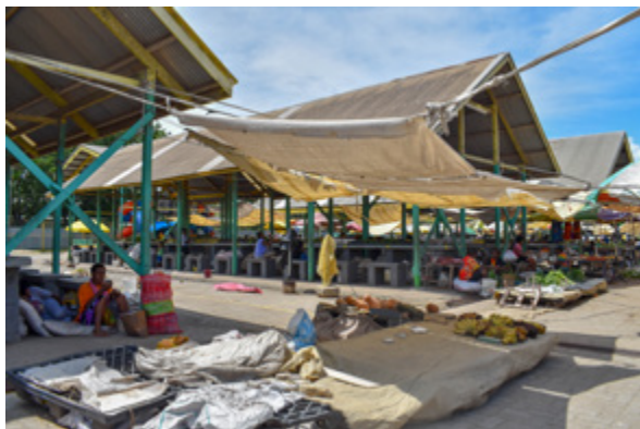
Gerehu market infrastructure (2018)
