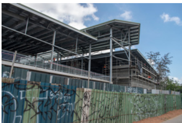
Gordons market under construction (2018)
